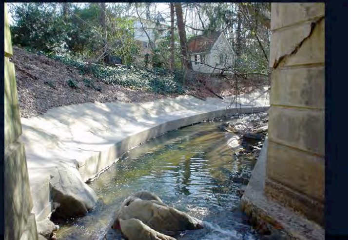
Up Stream along Goldsboro between MacArthur Blvd and Tulip Hill
